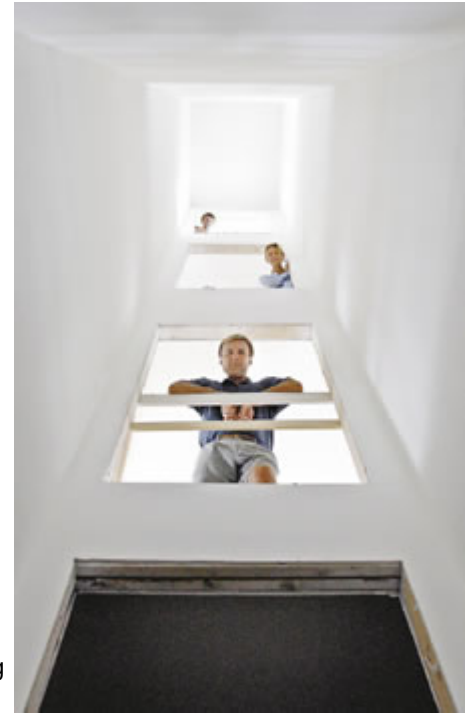
Paul Klinefelter, on first level, wife Sue Anne, and son Daniel, top level, plan on using the elevator in their new Goochland County home to move furniture from one level to another. The house is being built by Pitts & Associates.
