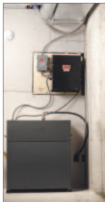
The operating hardware of Cambridge Elevating's residential elevators.
